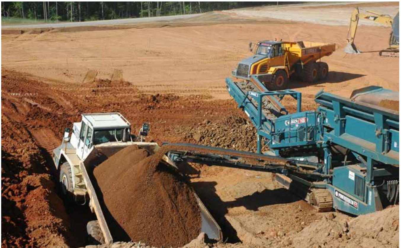
Figure 46. On-site grinding and blending of a planting soil material
