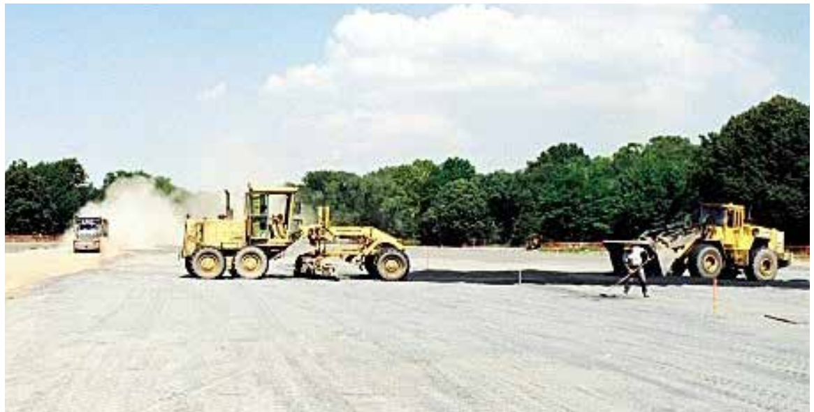
Figure 47. Spreading structural soil at Great Lawn in Central Park, New York, NY
